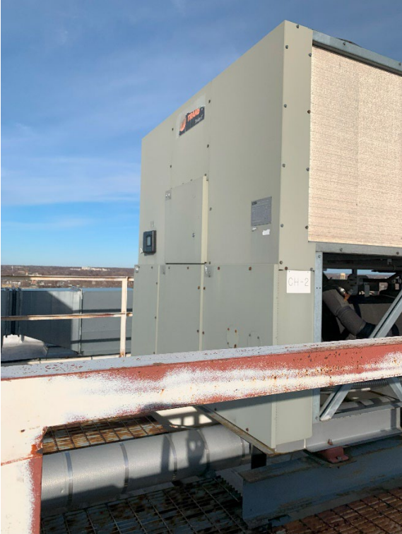
Figure 25: Courthouse Roof Top Chiller CH-1 and CH-2 Control Panels
