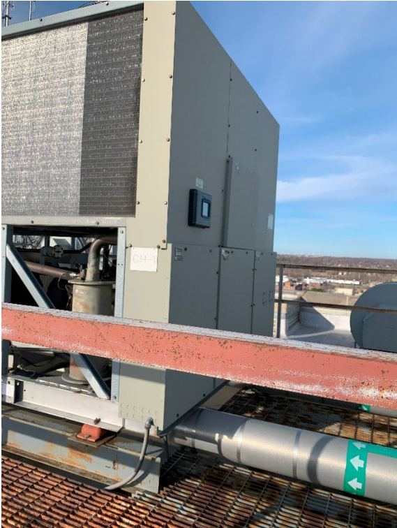
Figure 25: Courthouse Roof Top Chiller CH-1 and CH-2 Control Panels
