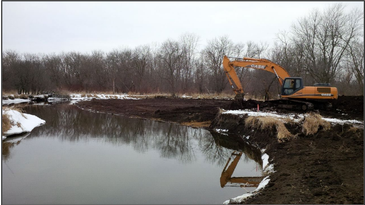
Photo 4: Grading bank to mimic natural slopes and morphology at Nippersink Creek, IL
