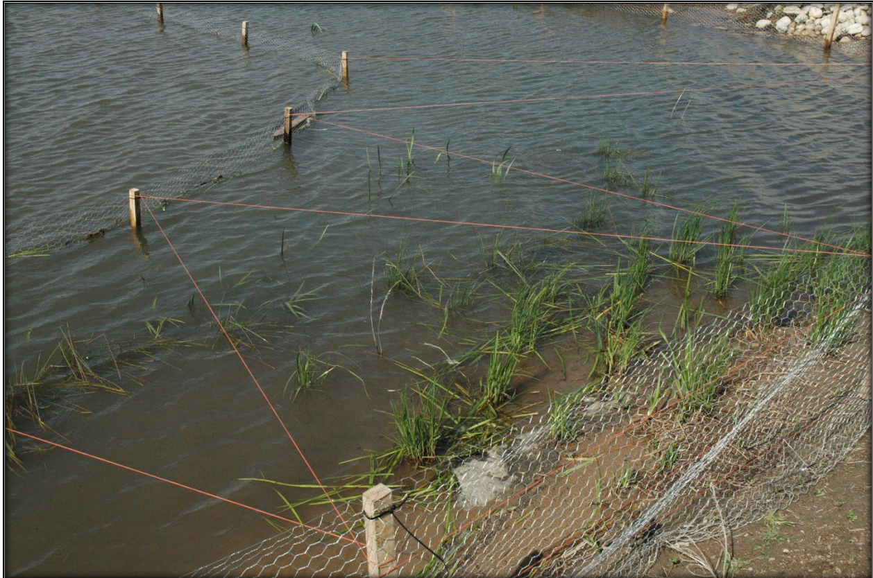
Photo 8: Common Carp and Canada geese protection for newly planted wetlands plugs
