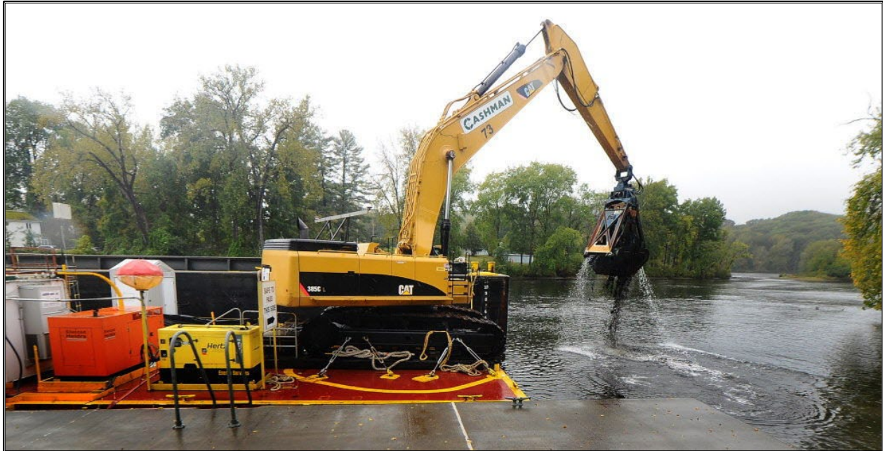
Photo 3: Mechanical riverine dredging of sediments, USEPA
