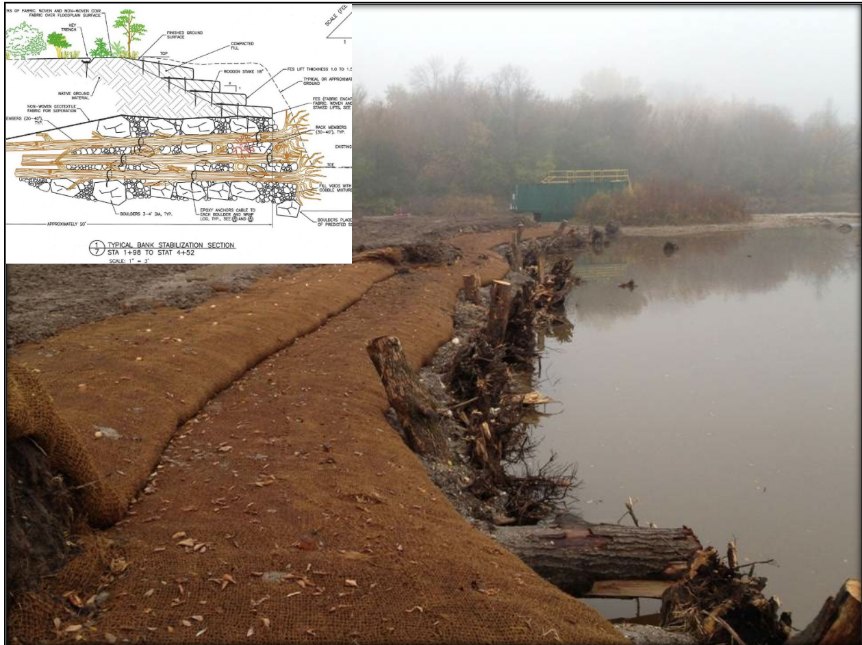
Photo 6: Large woody debris structure and soil terracing
