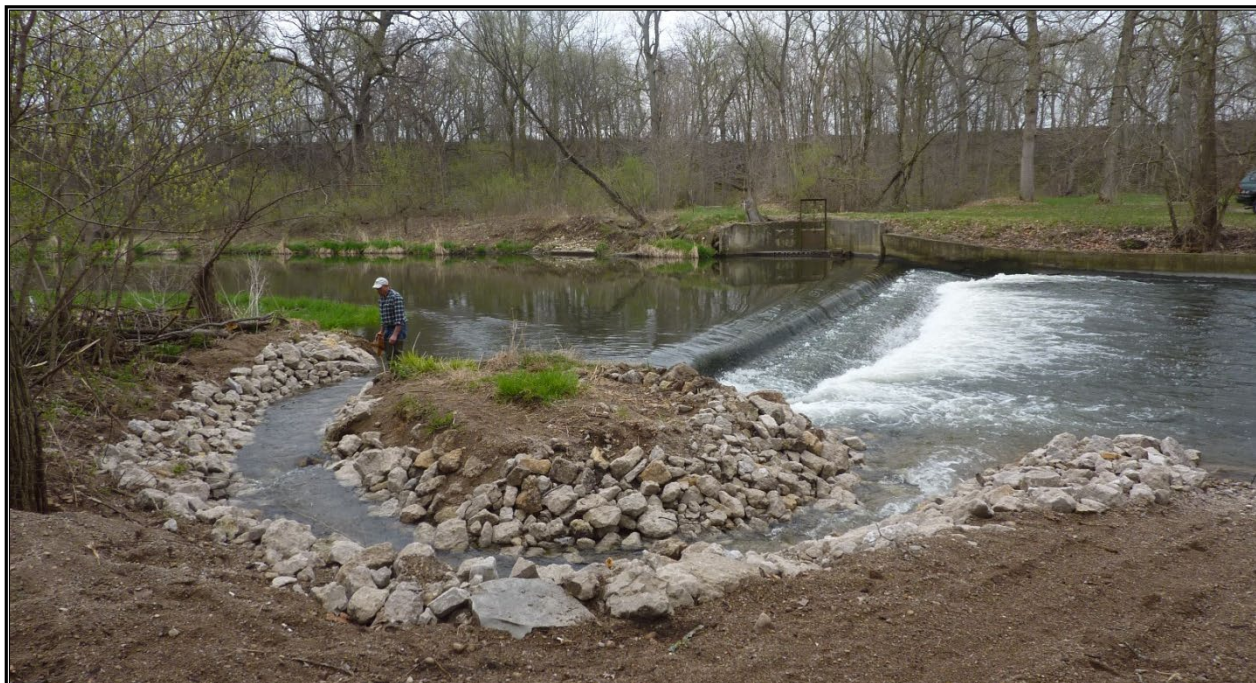
Photo 2: Bypass channel on Big Rock Creek, IL
