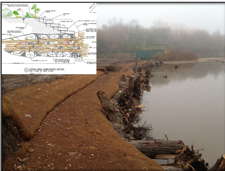
Photo 6: Large Woody Debris Structure and Soil Terracing, AER
