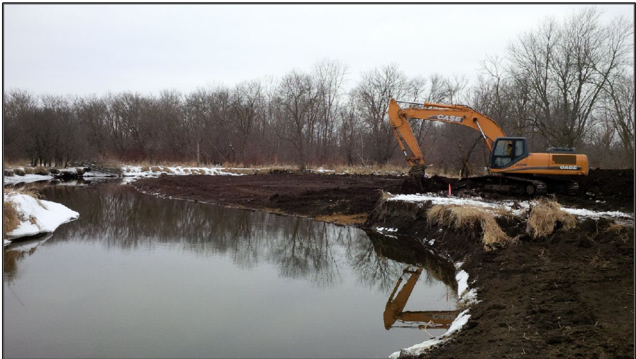
Photo 4: Grading Bank to Mimic Natural Slopes & Morphology at Nippersink Creek, AER
