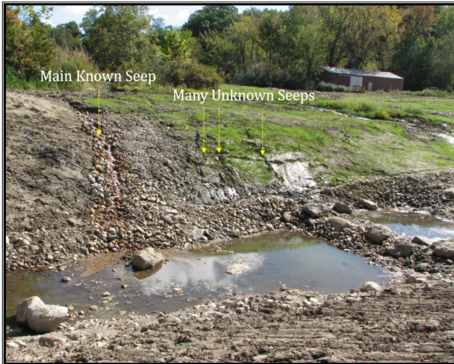
Photo 9: Adaptive Management of Seeps 1 st and 2 nd Year of Construction Red Mill Pond AER
