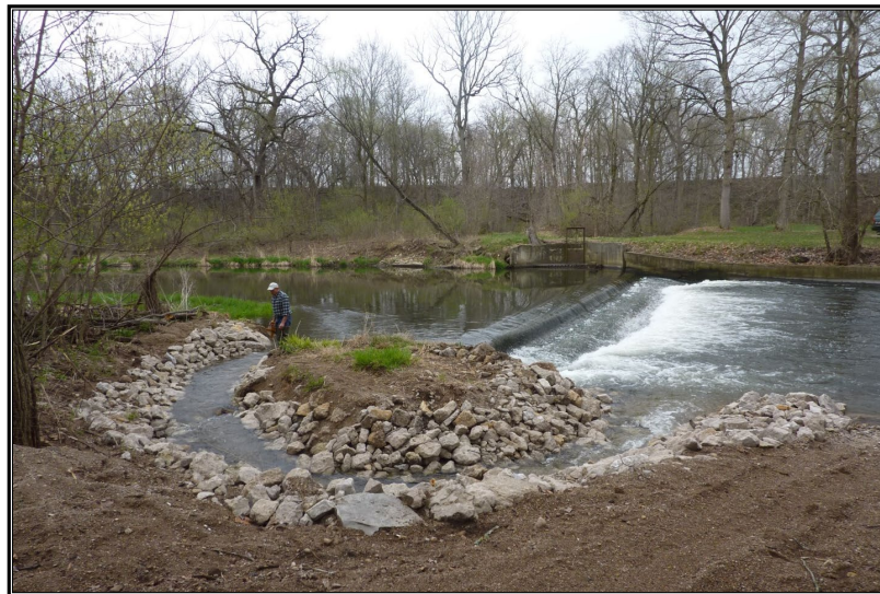
Photo 2: Bypass Channel on Big Rock Creek, Kendall County, IL
