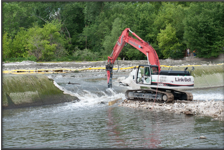
Photo 1: Demolition of the Hofmann Dam, AER
