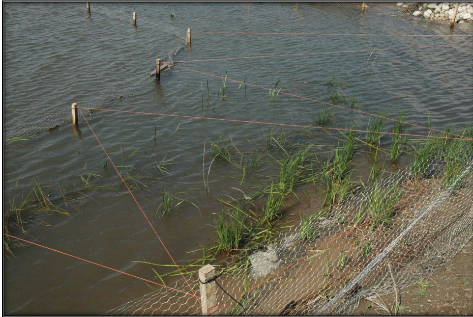
Photo 8: Common Carp and Canada Geese Protection for Newly Planted Wetlands Plugs, AER
