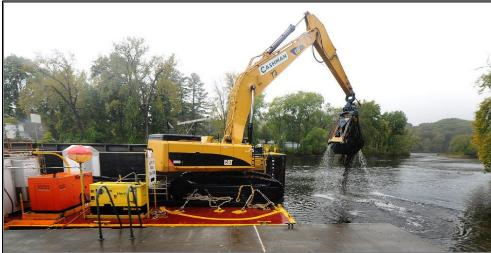
Photo 3: Mechanical Riverine Dredging of Sediments, USEPA
