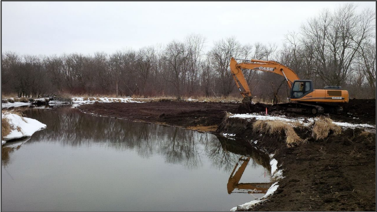
Photo 4: Grading bank to mimic natural slopes and morphology at Nippersink Creek, IL
