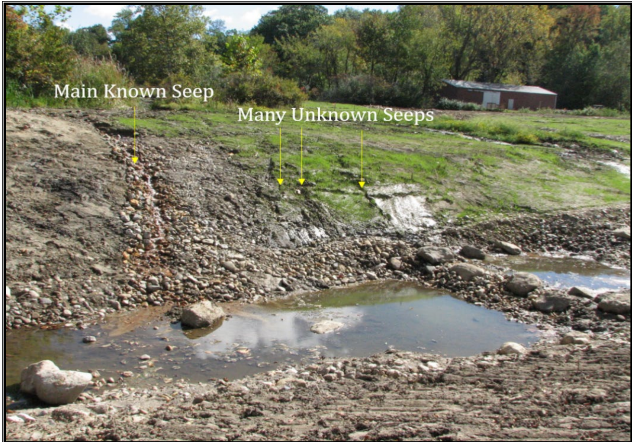
Photo 9: Adaptive management of seeps during construction at Red Mill Pond, IN
