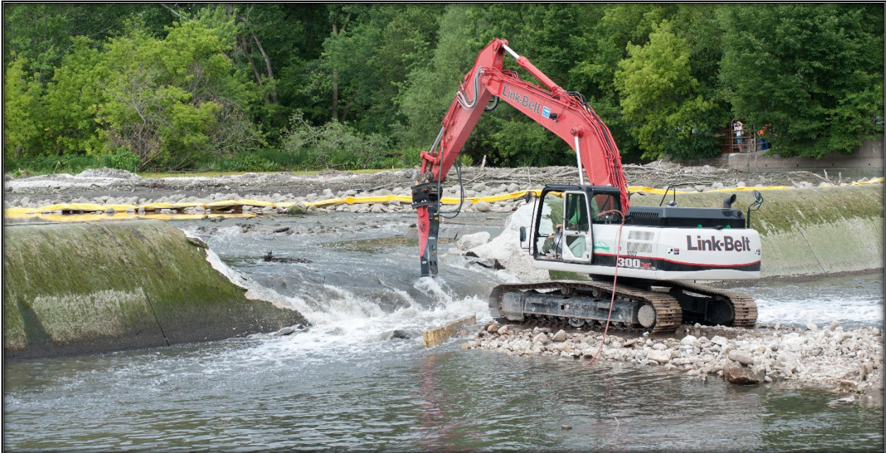
Photo 1: Demolition of the Hofmann Dam, IL
