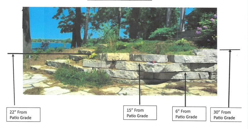
The Soil Retention wall is constructed from outcropping stone (approximately 7" thick) without any interlocking joints, glues and mortars. The overall Length is approximately 15 feet with a maximum height of 30 inches. Note the hill and grade was present prior to the wall.
