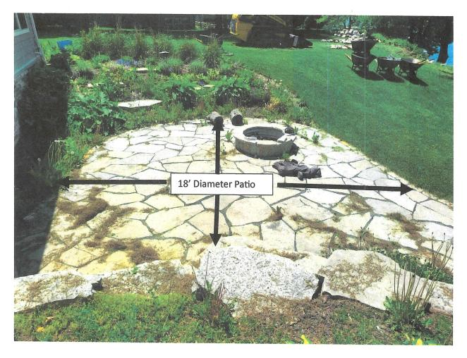
The Patio is constructed from flagstone with no grade change. Patio has the basic shape of a circle with a few transitional areas. The patio is npt connected to the house and is free floating.
