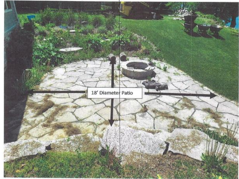
The Patio is constructed from flagstone with no grade change. Patio has the basic shape of a circle with a few transitional areas. The patio is not connected to the house and is free floating.
