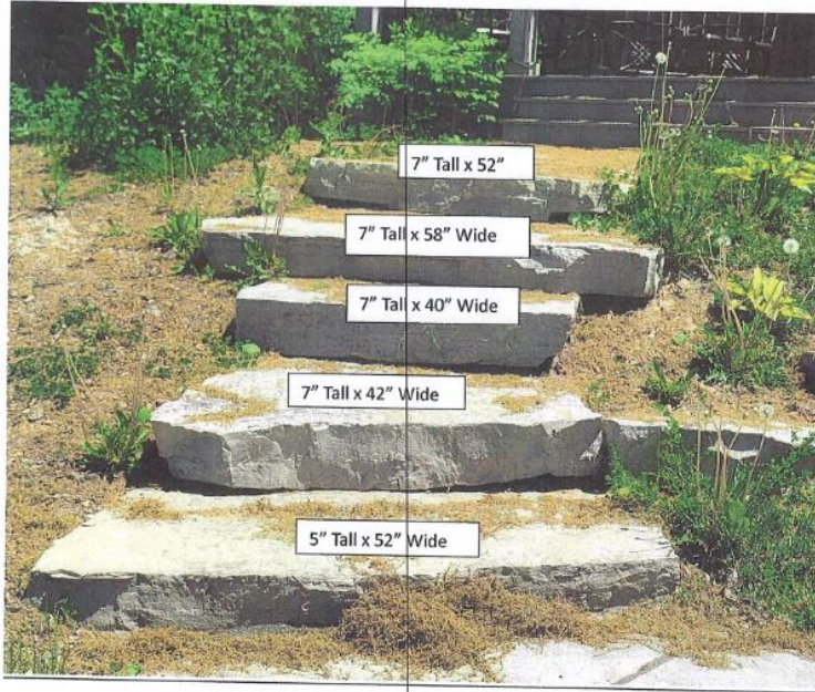
Detail "A" Outcropping Stone Steps to Deck
