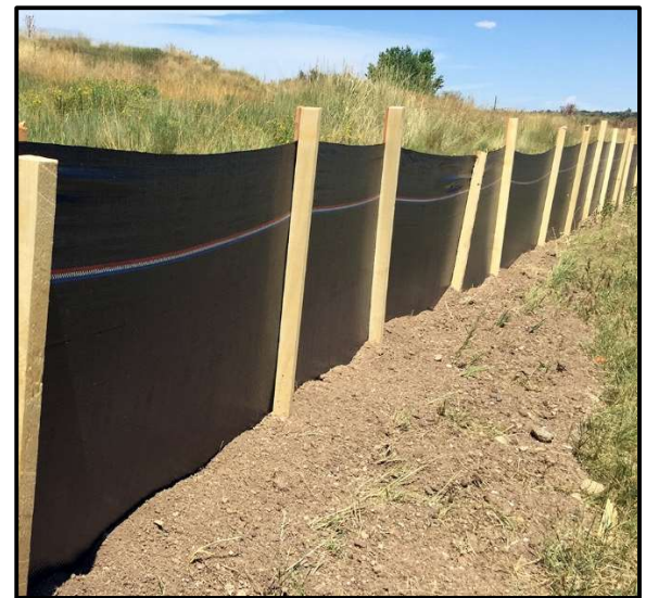
PROPERLY INSTALLED SILT FENCE.
