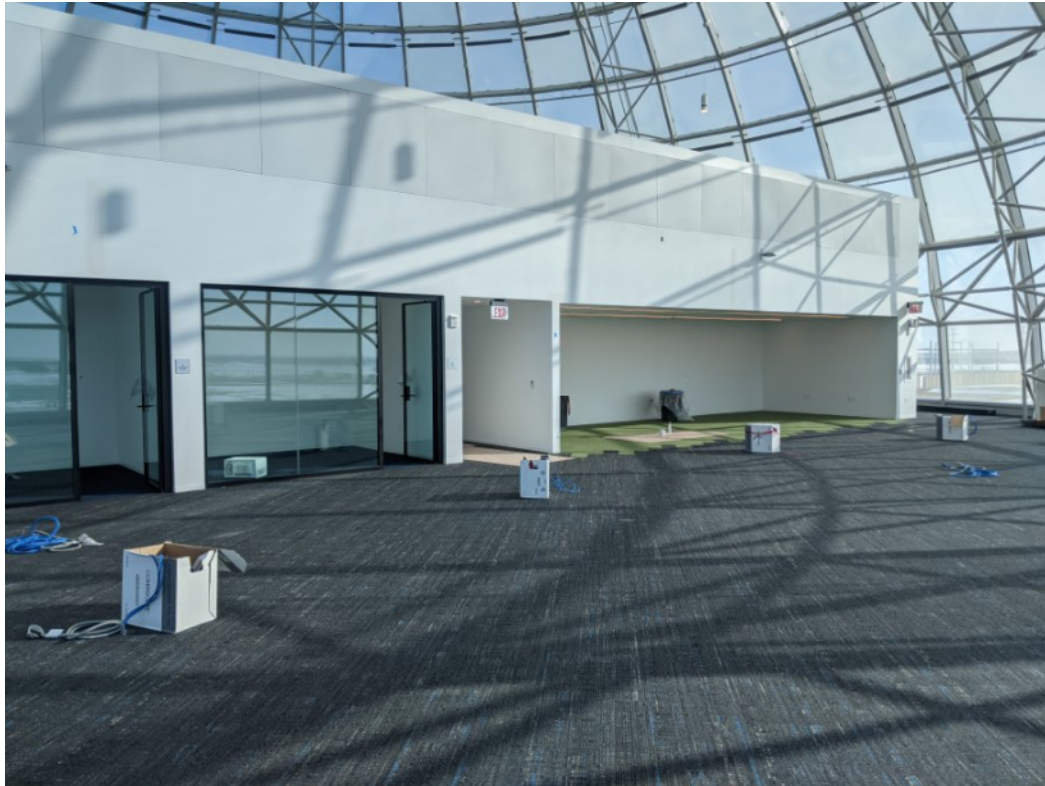
Complete drywall, painting and flooring installation on Level 3
