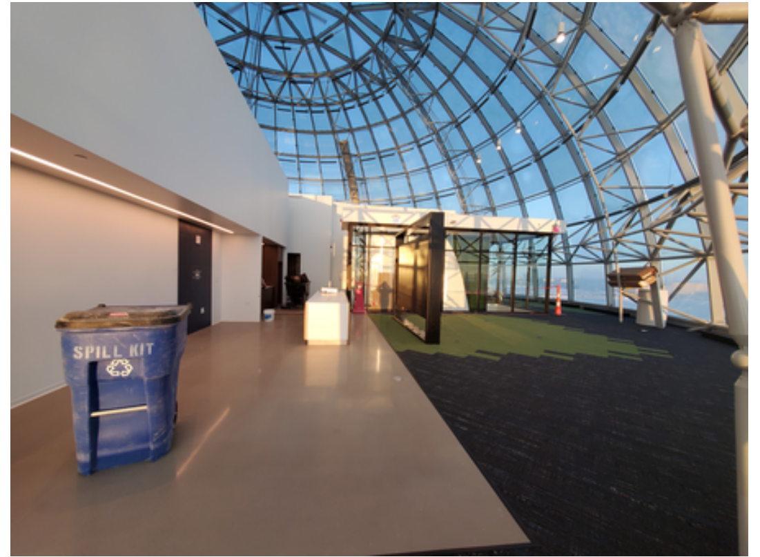
Completion of Level 3 concrete floor polishing
