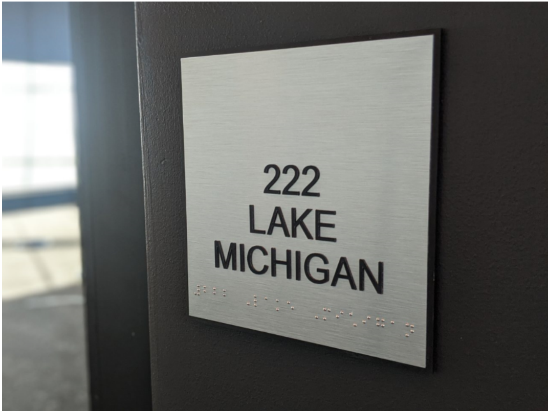
Complete installation of interior signage throughout the building
