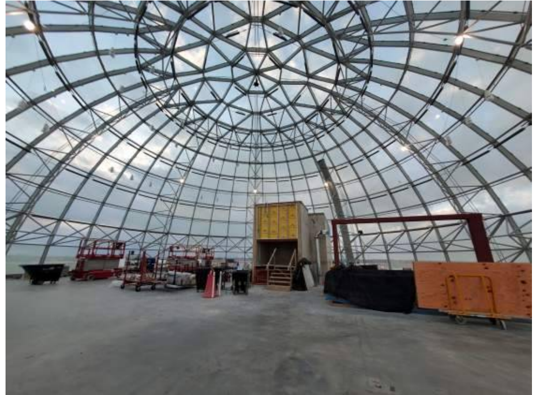
MEP Systems and Light Fixture Installation on the Domed Structure
