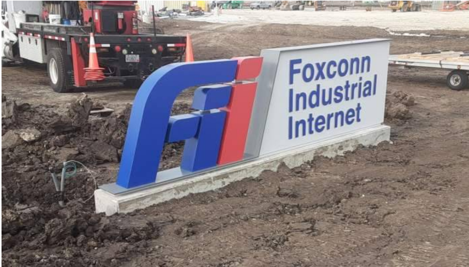
Installation Complete of the Exterior Monument Sign
