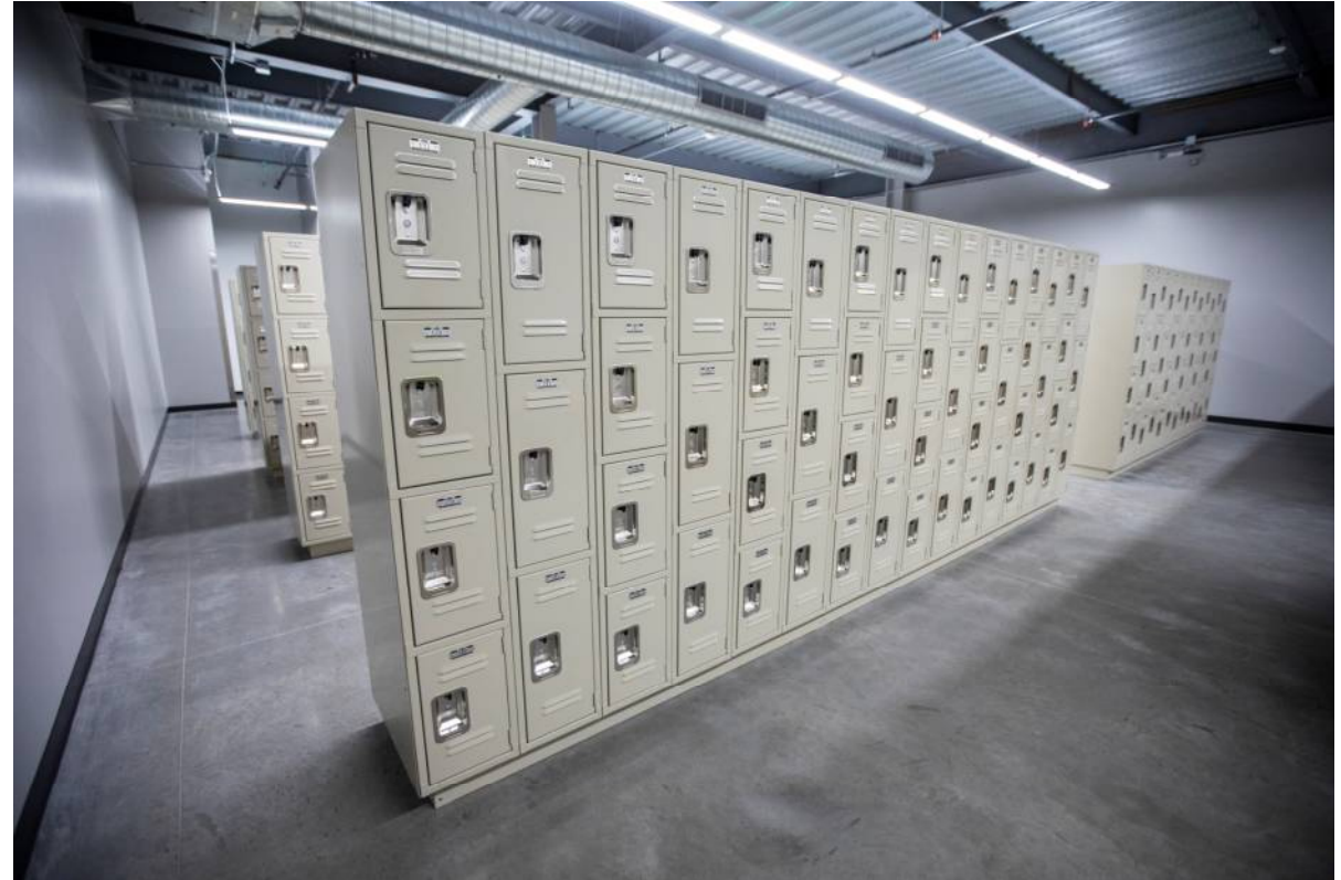
North Locker Room
