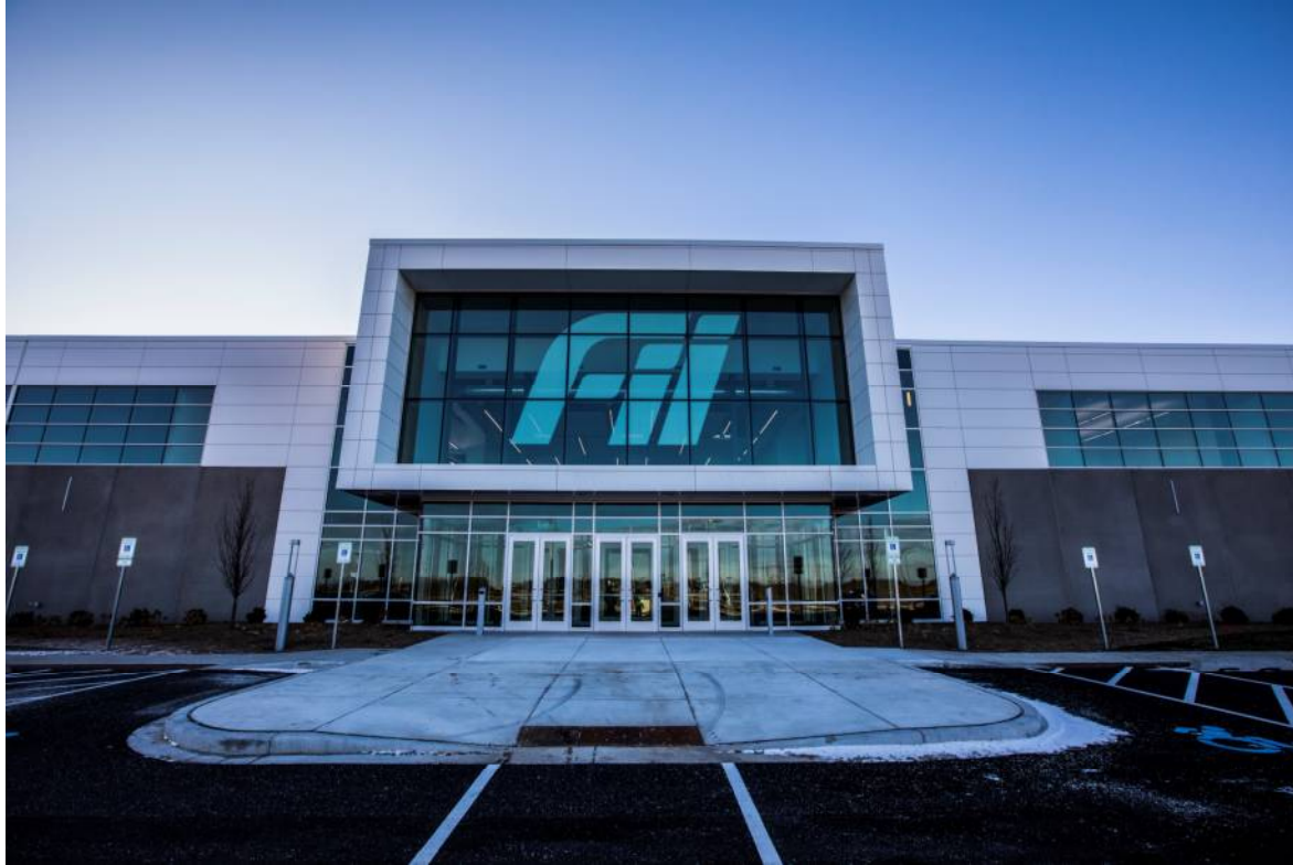
Exterior Front of Building
