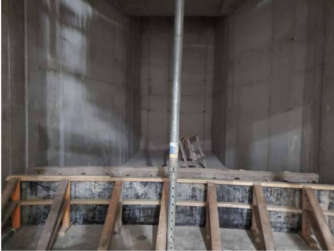
Intake Area Well Interior
