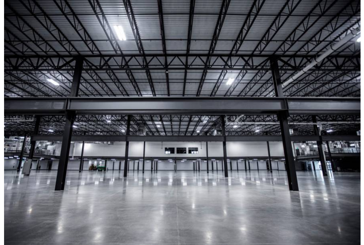
East Manufacturing Area
