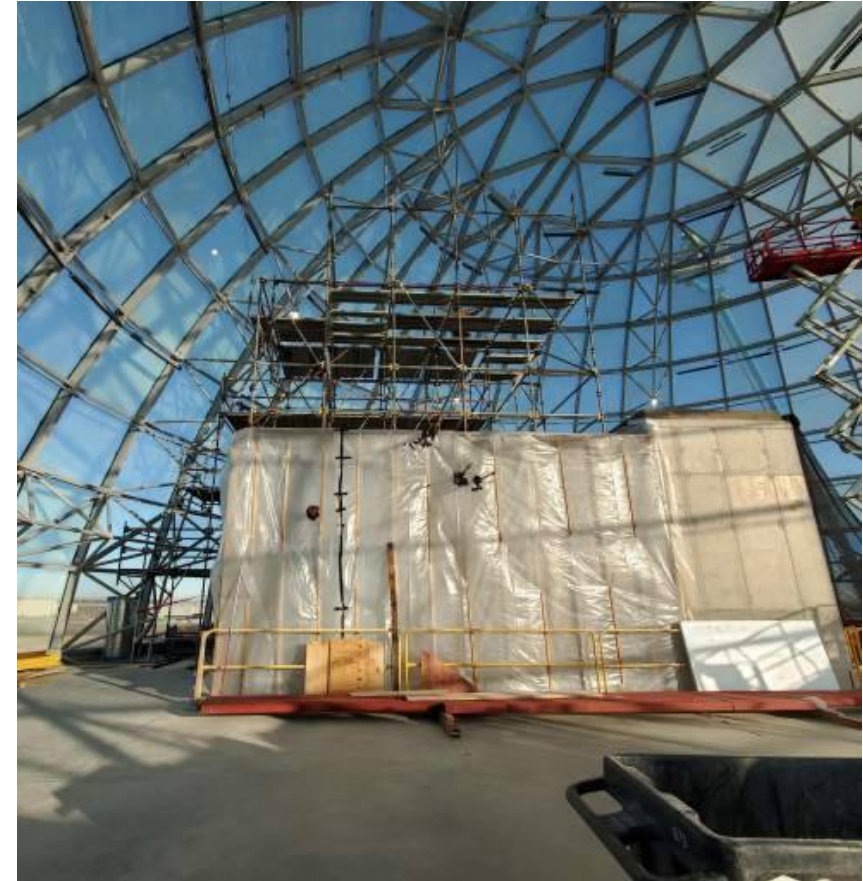
Begin Framing on the Third Floor
