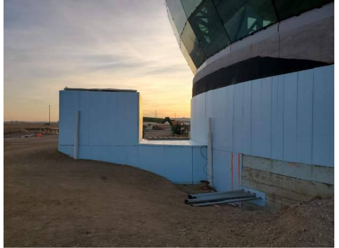
Waterproofing of Intake Area Well
