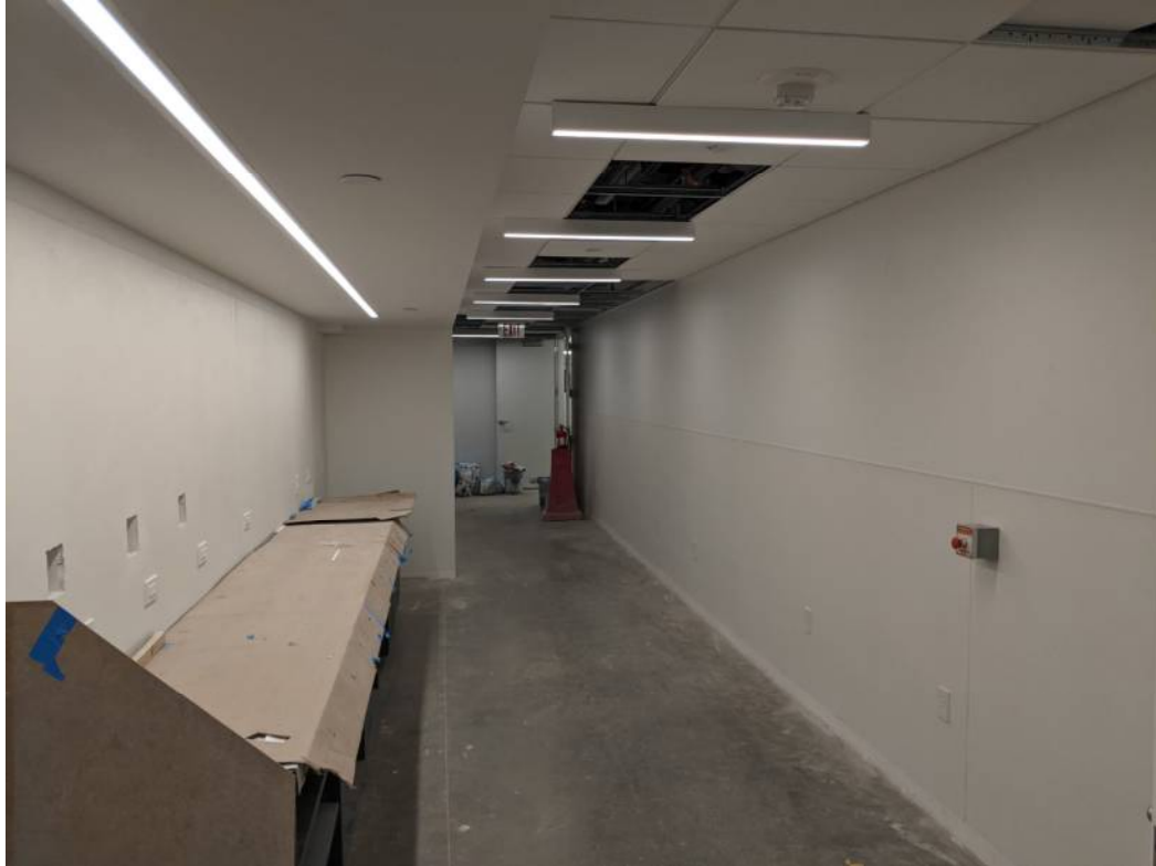
Begin painting and complete lighting installation in Lobby in Lower Level
