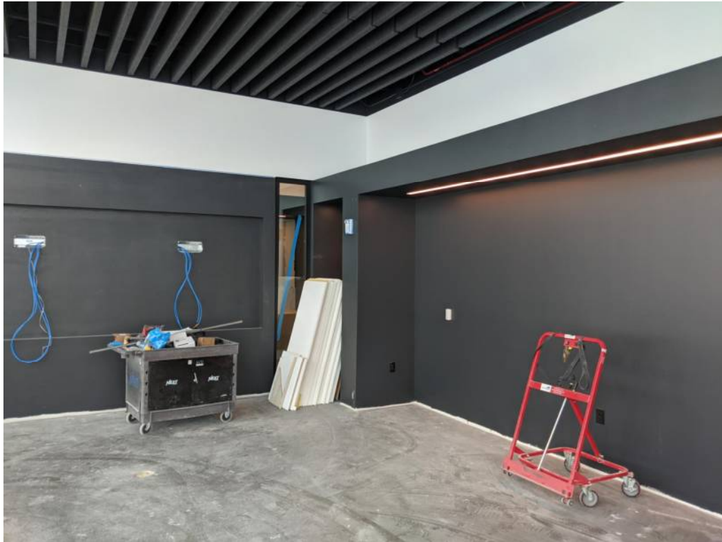
Continue painting and baffled ceiling installation in Level 2 Board Room
