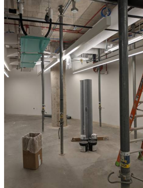
Begin painting in 5G R&D Room in Lower Level
