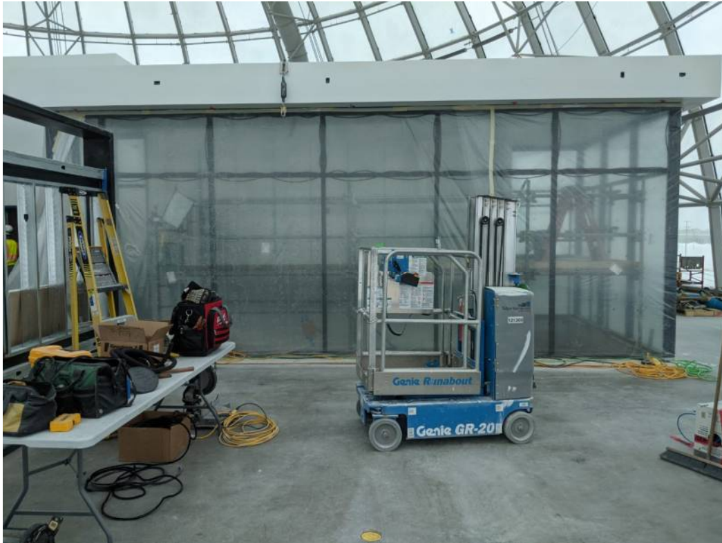
Begin painting and glazing installation of monument stair enclosure on Level 3
