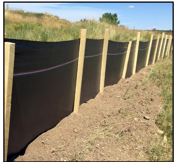
PROPERLY INSTALLED SILT FENCE.
