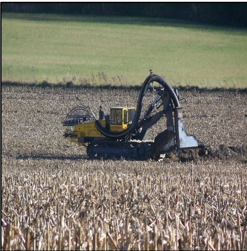
Installation of Drainage Tile
