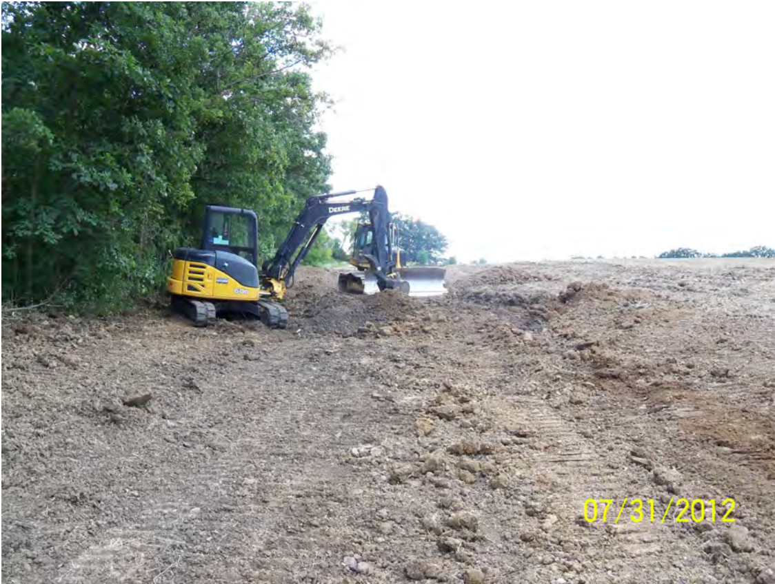
EXCAVATOR AND BULLDOZER GRADING IN THE GRASSED WATERWAY #2403
