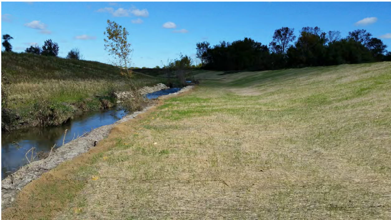
Construction completed with riprap on potential streambank erosion and erosion netting
