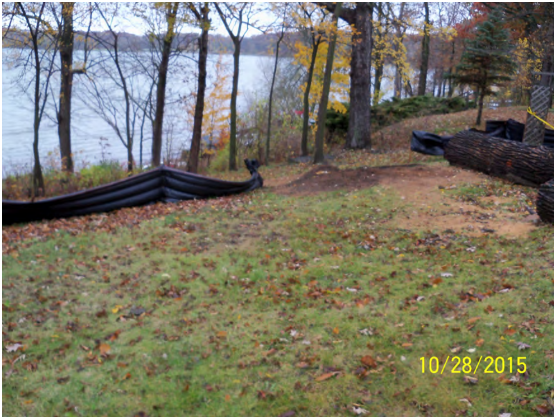
Silt fence improperly installed on Eagle Lake, not closed at the hill bottom.
